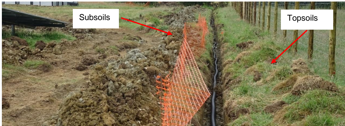
Insert 32: Subsoils Dug out of the Trench
